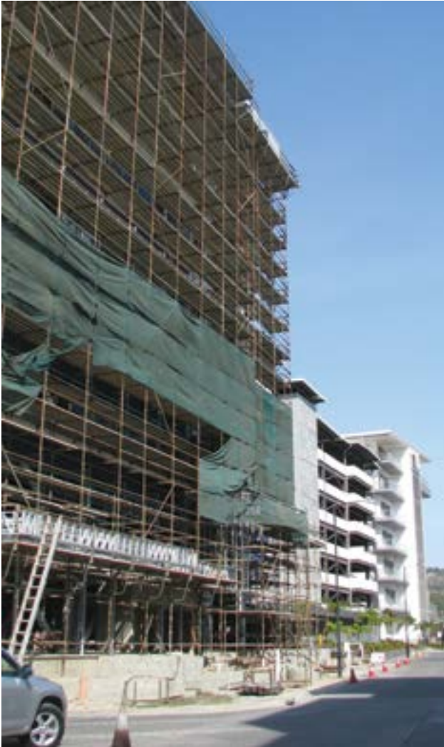
Construction at Port Moresby's Harbour City development continues apace.
