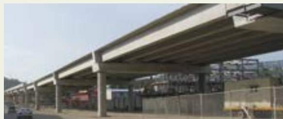
The Kookaburra Flyover under construction.
