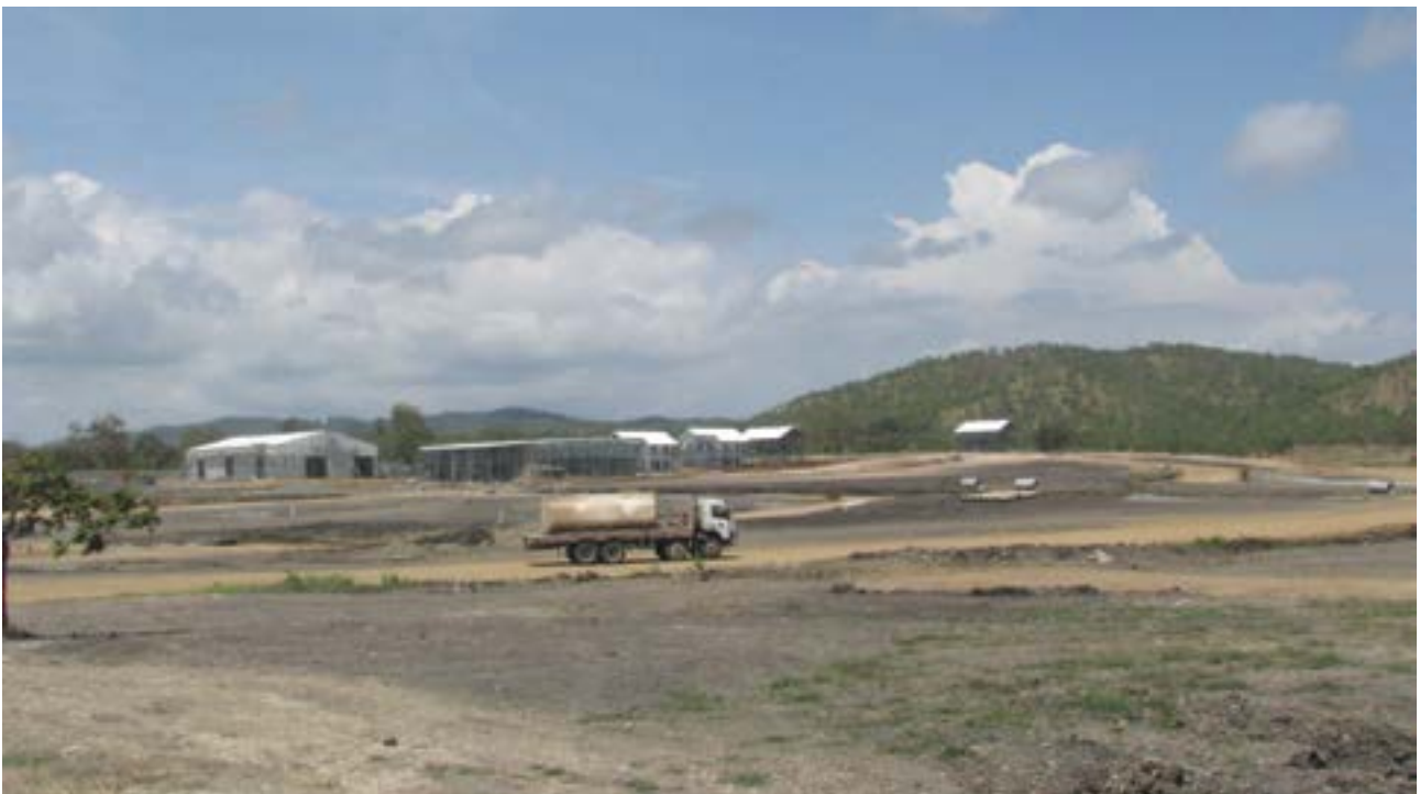
Edai Town, a contemporary, gated 500-unit executive K250 million (US$100 million) housing estate is under construction in Central Province. The township is part of a residential and logistics corridor between PNG's capital city and ExxonMobil's LNG Plant, 20 km north-west of Port Moresby.
