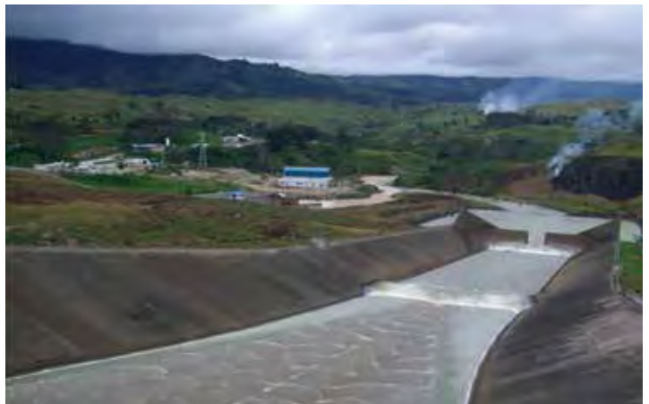
The Yonki 'Toe of the Dam' hydroelectric project in Eastern Highlands Province. PNG Power
