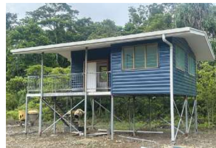
Families from one village on Woodlark Island have agreed to be relocated into new steel-framed homes, to allow for the development of three planned open pits.
