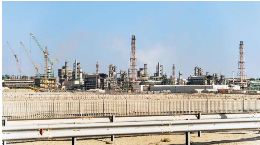
Gas production facilities in Qatar, the world’s largest LNG exporter. An Iranian missile strike in March 2026 removed around 17 per cent of the country’s gas exporting capacity.
