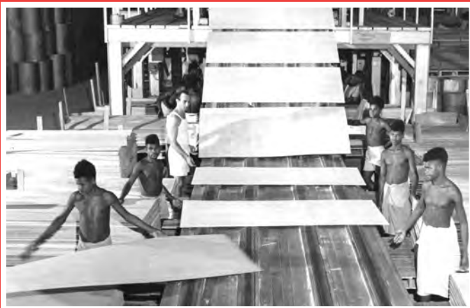
Nation building (from top): a Junkers aircraft involved in the development of Bulolo; PNG Forest Products bridge building; TE PNG techs at work; an early plywood mill.
